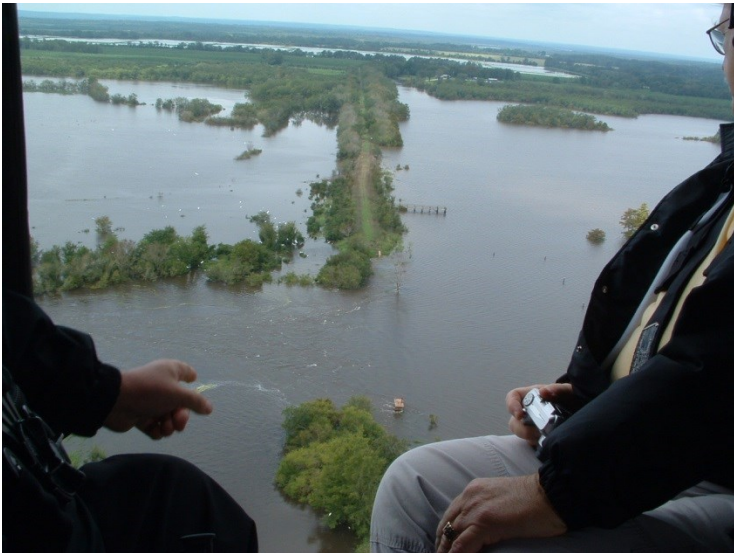
Northeast Louisiana, post-Gustav, from the Blackhawk. Water is only supposed to be on the right-hand side of the levee...
